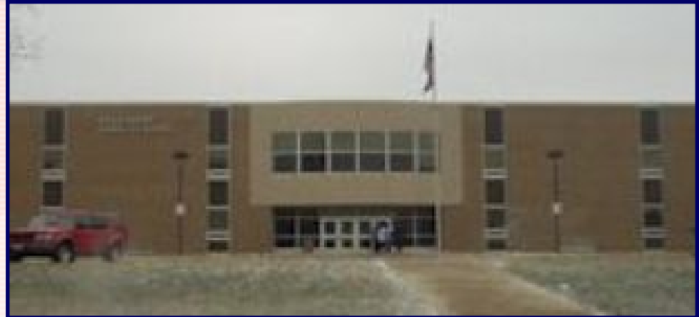
Belvidere High School, photo courtesy of district100.com
